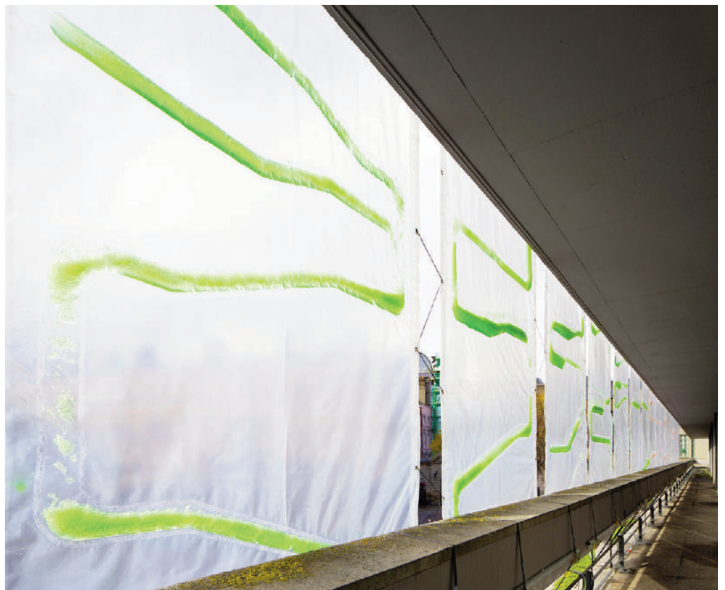
Fig. 8-10 | Photo.Synth.Etica. An urban tent that captures carbon dioxide and releases oxygen thanks to the beneficial acts of micro-algae. A bio-tent envelops the first and second floor of the main facade of the Printworks Building at the Dublin Castle and is composed of 16 modules, each measuring 2 x 7 meters. The proposal suggests the use of cutting-edge technology based on digital and biological intelligence as a potential avenue to addressing the issue of urban design. Architect: ecoLogicStudio (C. Pasquero, M. Poletto); Design Team: K. Alexopoulos, N. Aulitzky, S. Soni, R. Staples, C. Vrantzi, C. W. Yang; Structural Engineering: M. van de Worp – Nous Engineering, USA; Bioplastic Supply and Manufacturing Support: J. Woollard – Polythene, UK; Microalgae Cultures Supply: Dr. Fiona Moejes – Bantry Marine Research Station, Ireland (photos by NAARO).
