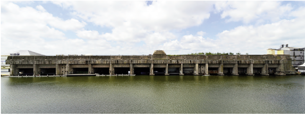
Fig. 1 | The submarine base of Saint-Nazaire, Alvéoles 12-14 (source: commons.wikimedia.org, 2012).
