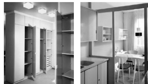
Figg. 6, 7 - Model of apartment Neues Lebenneues Wohnen (W. Stallknecht, 1963) in Berlin: the glass door as an alternative to the door and the cabinets as an alternative to partitions; Example of apartment distribution (W. Stallknecht, 1982), conceived by the residents themselves, from light partitions or from furnishing elements (credits: W. Stallknecht).
