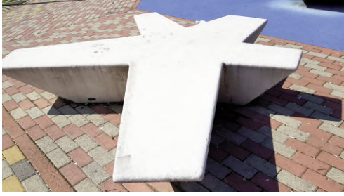
Fig. 8 - Flor, manufactured by Escofet. Playground furniture made of self-compacting reinforced concrete with acid-etched waterproof finishing: colour variation, patina in lower area, staining, and local graffiti (operating life: 4 years); Parco Mennea, Turin (credit: R. Maspoli, 2019).
