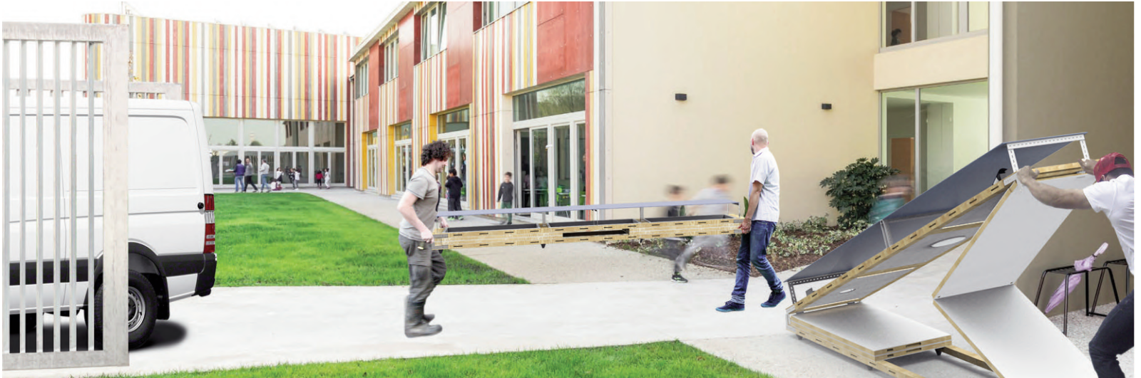
Fig. 10 - Transport and assembly of Merlino modules.
