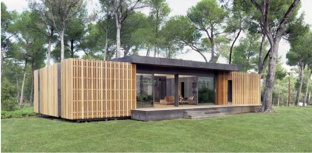
Fig. 4 - Pop-Up House: the passive house is ready in 4 days (credit: www.ingenio-web.it/3239-pop-up-house-la-casa-passiva-pronta-in-4-giorni ).
