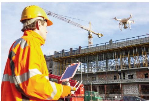
Fig. 9, 10 - Robotics applications (credit: www.bioedil-progetti.com/robot-costruira-case-digitalizzazione-edilizia/ ); Drone on construction site (credit: Kalinovsky.it.depositphotos.com/202239006/stock-photo-drone-operated-by-construction-worker.html ).
