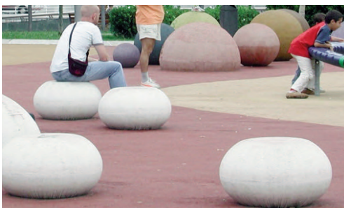
Fig. 5 - Monolith urban furniture benches made of concrete containing fine aggregates and with superficial etching and waterproof finishing: colour variation, slight patina in lower area (operating life: 4 years); Parco Nervion, Abandoibarra, Bilbao (credit: R. Maspoli, 2006).
