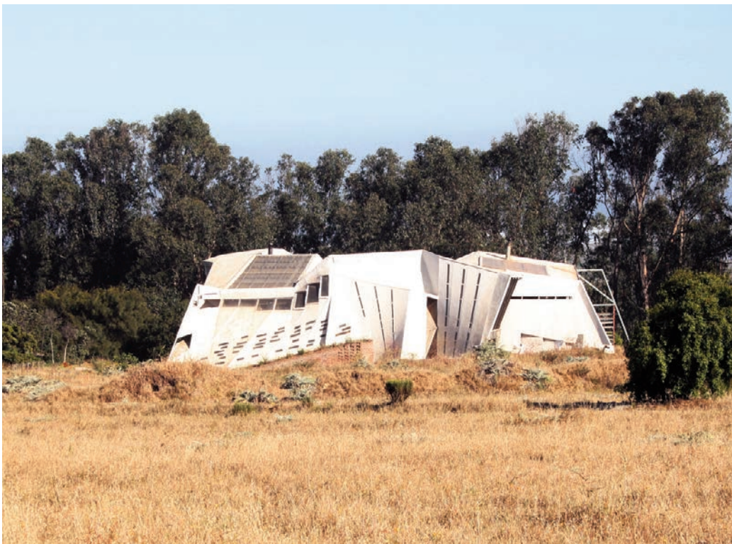
Fig. 4 - Hospedería del Errante, Open City, Ritoque (photo by Brighenti, 2013).
