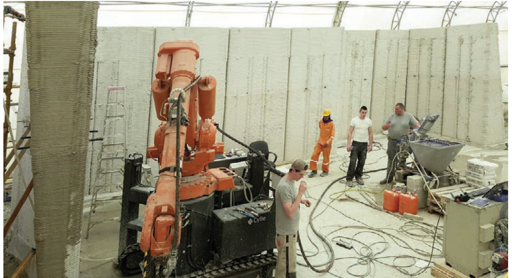
Fig. 9 - R&Drone Laboratory at Dubai building by a mobile 3D-printer, which is able to move on caterpillar tracks, for the construction of large buildings (photo by CyBe).
