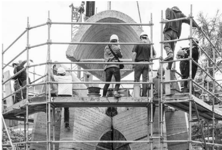
Fig. 2 - Spiro, A., "Department of Architecture, ETH Zürich", in Domus 1006 , 2016. Dome, made from prefabricated elements, designed and built by the students on the Höggerberg campus, during a workshop in 2014.
