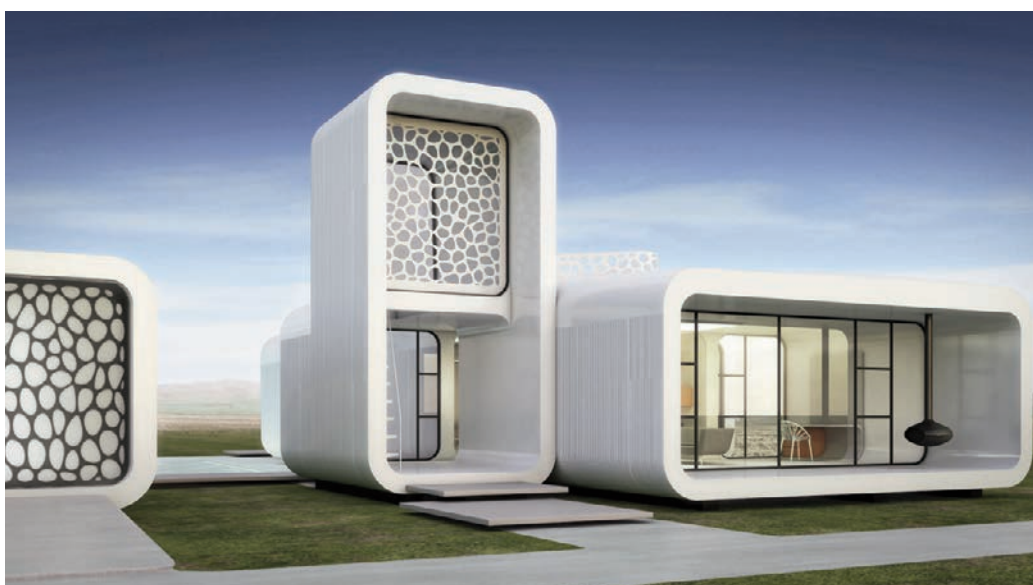
Fig. 13 - Pop up building (Dubai) 3D printed (photo by WinSun).
