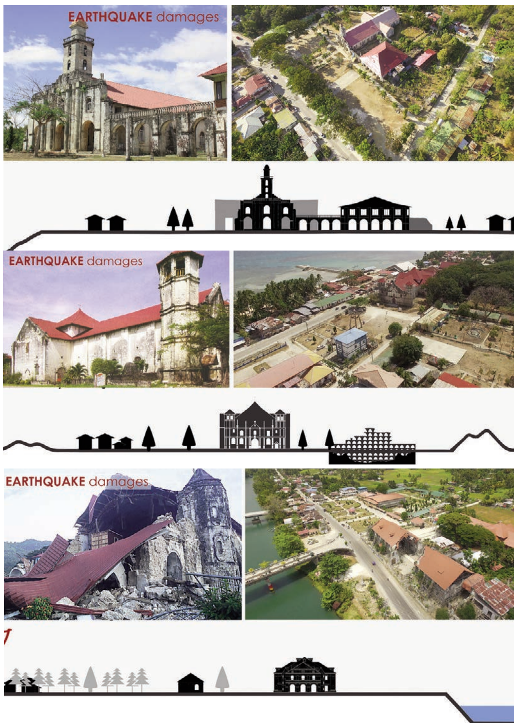
Fig. 2-4 - From the top: Post-earthquake damages in Santa Monica Church, Albuquerque, Bohol, Philippines (photos UPD's, drawings S. Schiazzano 2016); Post-earthquake damages in San Nicola Tolentino, Dimiao, Bohol, Philippines (UPD's photos, drawings F. Vardaro, 2016); Post-earthquake damages in San Pietro and Pablo, Loboc, Bohol, Philippines (UPD's photos, drawings A. Mustilli, 2016).
