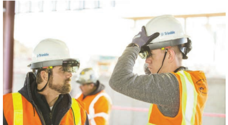
Fig. 2 - The augmented reality technology with the aid of viewers allows access to the project visualizing what happens on the construction site ( www.rivistageo.com/2018/01/27/10985/bim-cad-gis/trimble-ha-iniziato-a-rendere-operativa-la-mixed-reality-in-cantiere/ ).
