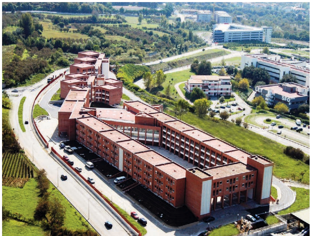
Fig. 15 - University Residence in Fisciano: aerial view of the residential complex (E. Sicignano, C. Sicignano, 2003).
