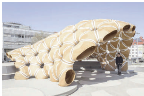
Fig. 1, 2 - Assembly Process, ICD Institute for Computational Design; Prof. Achim Menges, ITKE Institute of Building Structures and Structural Design; Prof. Jan Knippers, ICD/ITKE Research Pavilion 2015-16.
