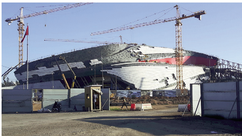
Fig. 5-7 | Grand Théâtre de Rabat (2010-2023) in Morocco, designed by Zaha Hadid Architects: The poetics of the object; Zoning related to the GRC façade panels; The laying of the skin (source: incide.co.uk).
