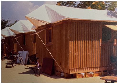
Fig. 6, 7 | The Paper Log House by Shigeru Ban in construction by volunteers (source: Christian, 2014).
