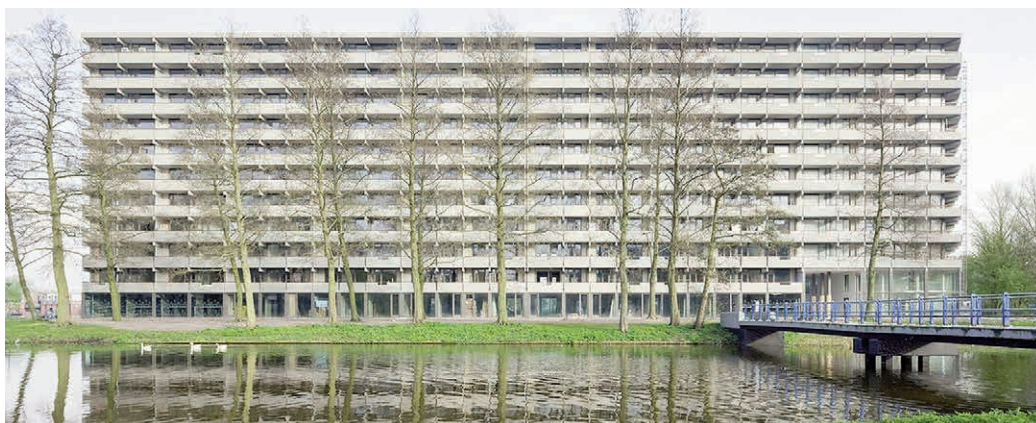
Fig. 6 | Deflat Kleiburg in Amsterdam, 2013-2016, designed by NL Architects and XWV architectuur (credit: M. Van der Burg, 2016).
