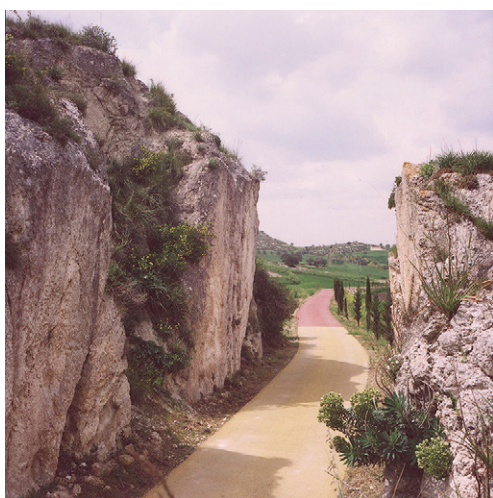
Fig. 6, 7 | Sections of the cycle-pedestrian path of the Linear Park between Caltagirone and San Michele di Ganzaria, designed by Studio NOWA (credits: Lotus Navigator; 2003).
