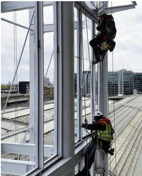
Fig. 8 | Installation of the first module of a structural bonding unitized system (credit: Focchi SpA, 2019).
