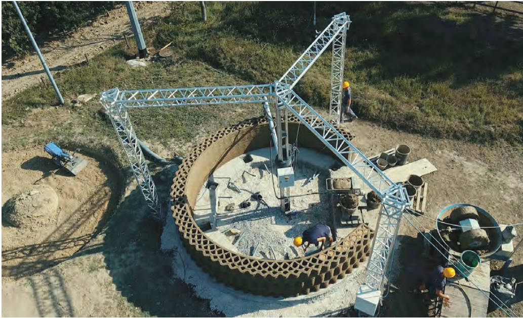
Fig. 1 | Gaia WASP | Crane 3D printed house (credit: WASP).
