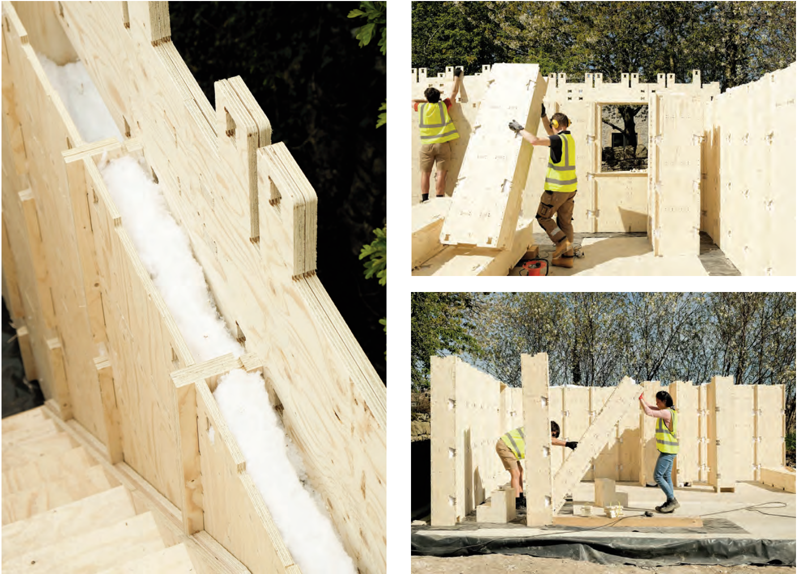
Figg. 2-4 | WikiHouse, a stage in assembling a prototype of the WikiHouse Skylark building system (credit: J. Watts, 2022).
