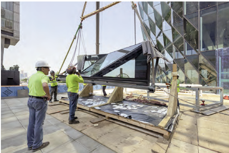
Fig. 5, 6 | Installation of the module of a 3D spatial system (diamond-like façade) in insulated double glass (credits: Focchi SpA, 2018).
