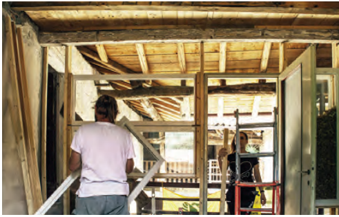
Fig. 8 | A phase of the Workshop of Thesis conducted in 2021 at Casamatta – Legambiente Varese, in Malnate (VA), AUIC School – Politecnico di Milano: the workshop envisaged the design and realisation of perimeter walls using reclaimed doors and windows and building components, identified in the area through the RE-sign platform (credit: M. Zanini, 2021).
