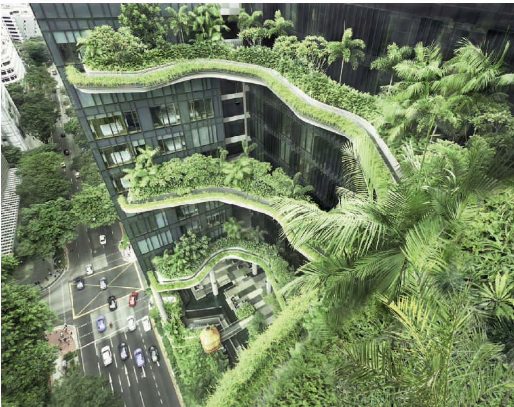
Fig. 15, 16 | Detail of the green roof installed in the basement part of the building, above a stratified artificial soil made of stepped moulded slabs; Detail of the green roof installed on the three cantilevered floors set between the building's avant-corps (credits: Patrick Bingham-Hall, WOHA).
