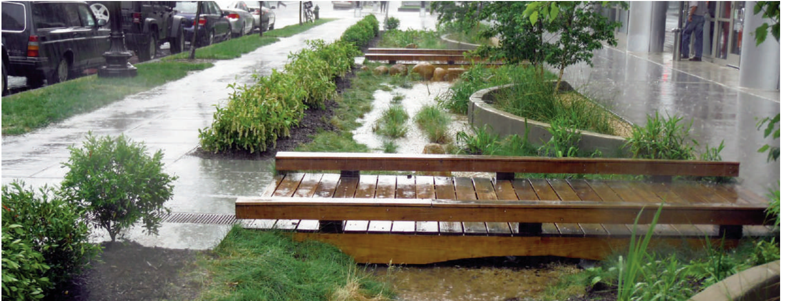
Fig. 11 | District Department of Energy and the Environment Headquarter, innovative curbside bioretention in the street right of way (credit: Prospect Waterproofing Co. – Green Roof, EcoSolutions – Bioretention, District Department of Energy and the Environment).
