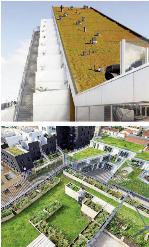
Fig. 4 | Examples of horizontal greenery systems: Bjarke Ingels Group, House 8, Denmark, 2010; Agence Engasser + Associés, 104 logements à Ivry-sur-Seine, France, 2017 (credits: J. Lanoo, 2010; M. Denancé and M. Ducros, 2017).
