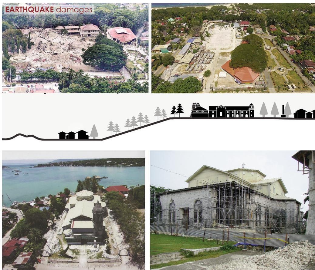
Fig. 5, 6 - From the top: Post-earthquake damages in Our Light Cathedral, Loon, Bohol, Philippines (UPD's photos, drawings F. Sommella, 2016); Post-earthquake damages in Our Lady Assumption, Dauis, Bohol, Philippines (UPD's photos, drawings).
