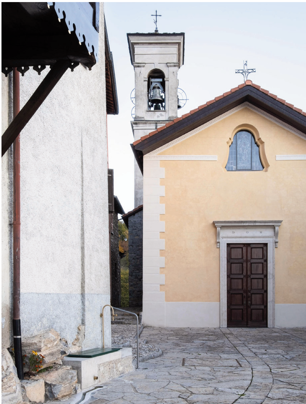
Fig. 4 | StudioSer introduced a new seating with an integrated fountain and gutter in the square in front of the church in Monte, once a site for congregation and play, to make it lively again, and more comfortable (credit: S. Högger, 2022).
