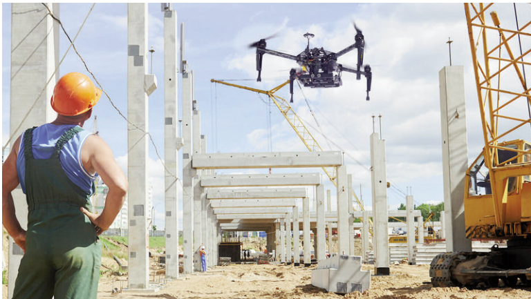
Fig. 1 - The use of drones facilitates risk analysis on site and ensures greater safety ( www.dronezine.it/40400/dagli-usa-cinque-lezioni-usare-droni-nelledilizia/ ).
