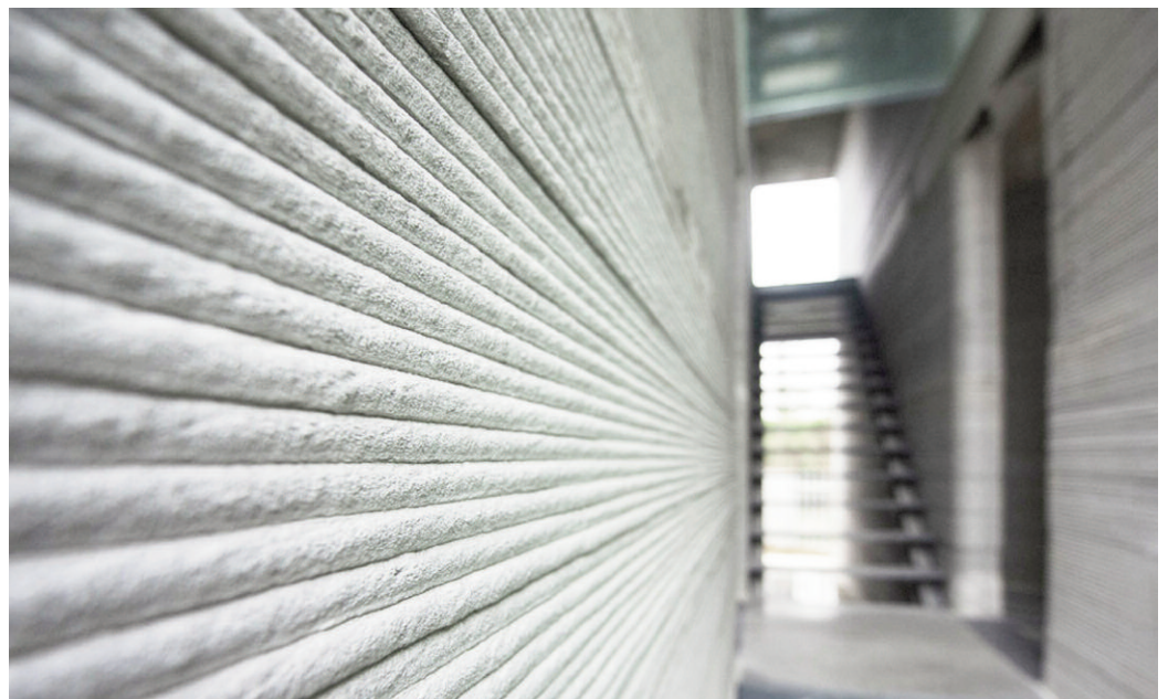
Fig. 10 - Concrete box, prints layer by layer with the typical texture (photo by WinSun).
