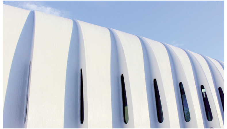
Fig. 11, 12 - AMIE (Additive Manufacturing Integrated Energy) – SOM and Oak Ridge National Laboratory partnership – the integrated system connects a 3D-printed polymeric mobile pavilion and vehicle to showcase a new approach to energy production, use, storage and consumption on site (photo by C. Jones); detail of the 3D printed pavilion AMIE (photo by Skidmore, Owings & Merrill, US Department of Energy's).
