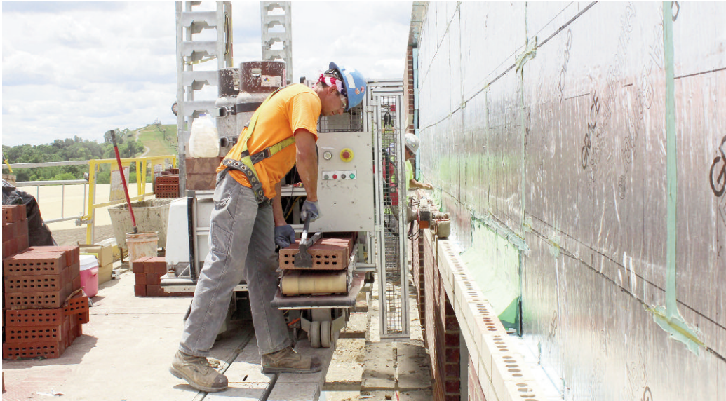
Fig. 7 - SAM/100 bricklaying robot, masons work together at the University of Michigan Brighton hospital (photo by Construction Robotics).
