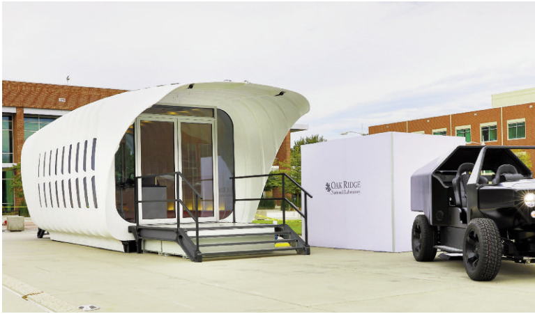
Fig. 11, 12 - AMIE (Additive Manufacturing Integrated Energy) – SOM and Oak Ridge National Laboratory partnership – the integrated system connects a 3D-printed polymeric mobile pavilion and vehicle to showcase a new approach to energy production, use, storage and consumption on site (photo by C. Jones); detail of the 3D printed pavilion AMIE (photo by Skidmore, Owings & Merrill, US Department of Energy's).
