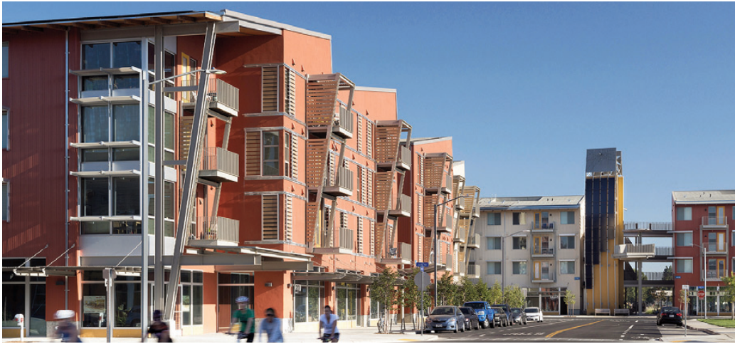
Fig. 1 | West Village (2013), University of California Davis (credit: Sherwin-Williams, 2015).
