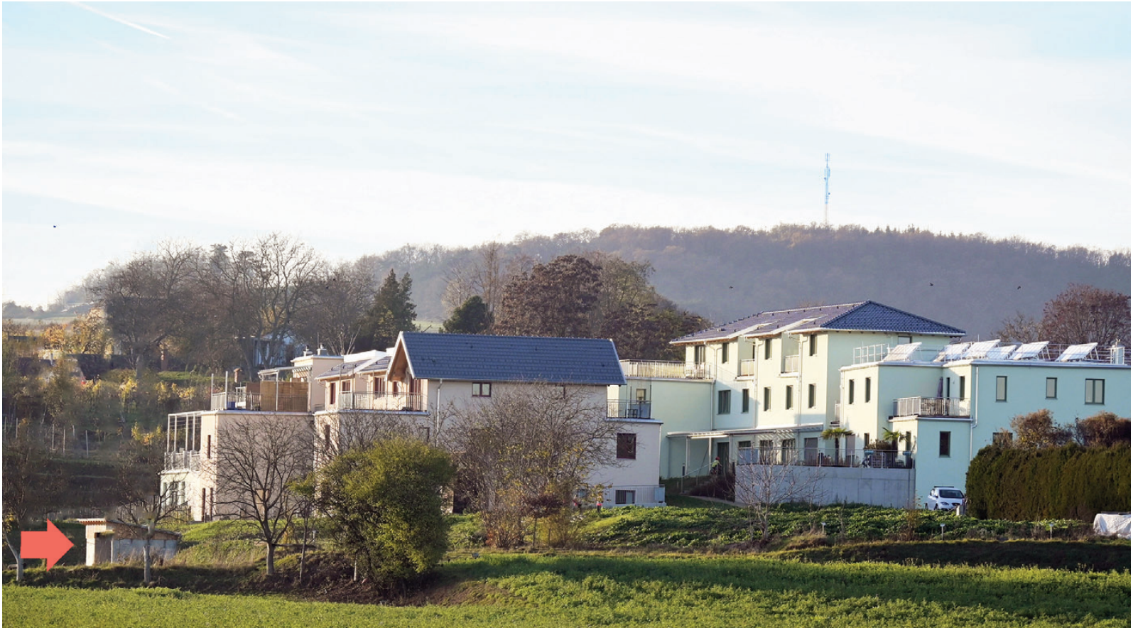
Fig. 35 | Social housing in Herzogenburg (Austria): the arrow on the bottom left indicates a small technical room housing two straw filters for wastewater treatment (credit: G. Mittersteiner, 2024).
