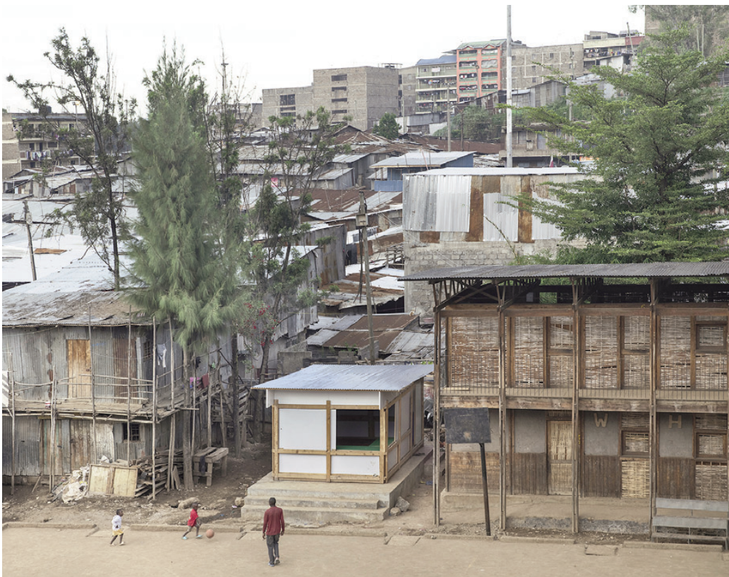
Fig. 29 | Canteen built in Nairobi by Giacomo Moor for the 2nd phase of the Design for Communities project: a homage to self-construction, the canteen is a micro-architecture designed to serve midday meals to school children (credits: F. Roman).
