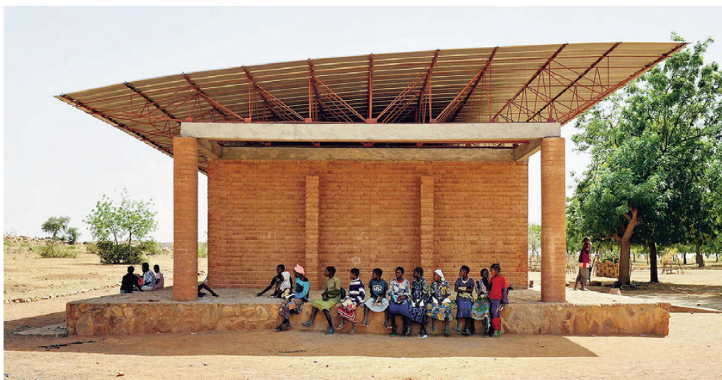
Figg. 1, 2 | Gando Primary School (2001) in southern Burkina Faso, designed by Francis Kéré: main elevation and building header (source: arquitecturaviva.com ).
