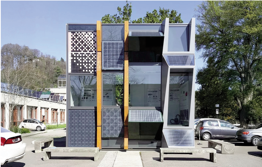
Fig. 1 | BIPV prototypes developed by the Institute for Applied Sustainability in the Built Environment research group at SUPSI (credit: SUPSI, 2021).
