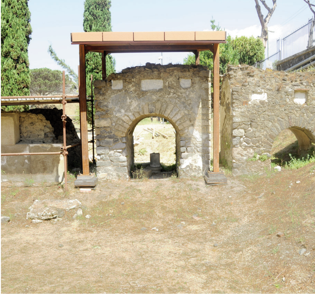
Fig. 8 | Reversible foundations, lead ballast elements (credits: R. Fonti, 2017).
