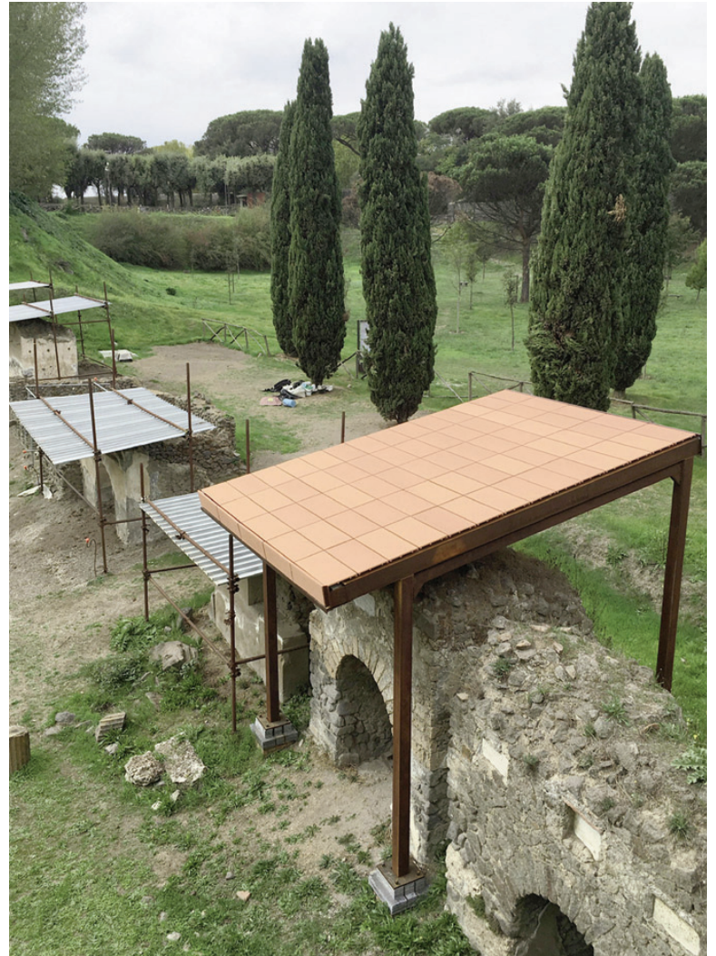
Fig. 7 | The prototype of protective shelter (credit: E. Emmerling, 2017).
