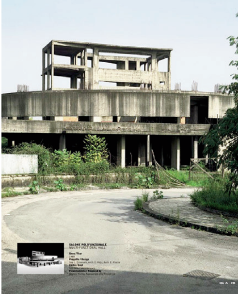
Fig. 24 | Unfinished multipurpose hall (1988) in Giarre (credit: G. Basilico).
