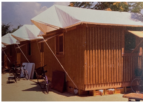
Fig. 6, 7 | The Paper Log House by Shigeru Ban in construction by volunteers (source: Christian, 2014).
