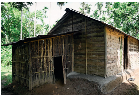
Fig. 9 | More recently, Better Shelter has been engaged in ways of filling the basic steel system of the Relief Housing Unit with local on-site materials, as is the case in Assam in India in 2023 (source: Better Shelter Organization, 2023).
