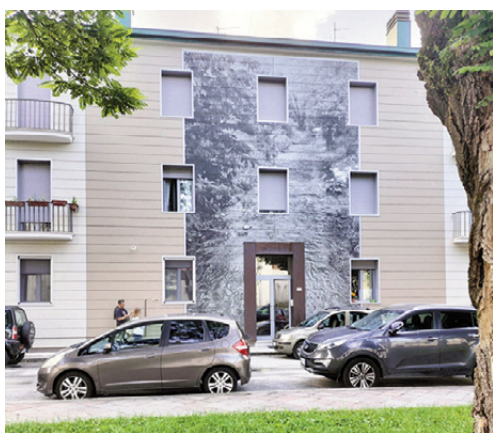
Fig. 10 | A Building in Castel di Sangro, central Italy (credit: P. Scala).
