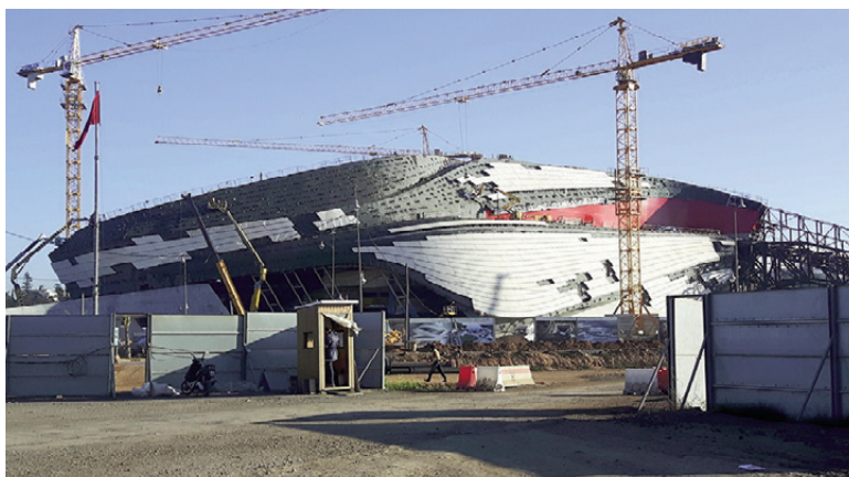
Fig. 5-7 | Grand Théâtre de Rabat (2010-2023) in Morocco, designed by Zaha Hadid Architects: The poetics of the object; Zoning related to the GRC façade panels; The laying of the skin (source: incide.co.uk).
