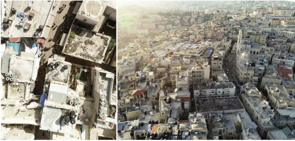
Fig. 1 | UAV photographic images of Bethlehem's Old Town showing the morphological complexity of the urban settlement (credit: '3D Bethlehem' Project, E. Doria, 2022).
