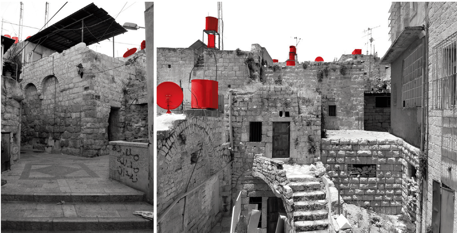
Fig. 4 | The cisterns on buildings in the historic center, highlighted in red; the photographs were taken from the ground and show how cisterns are strongly characterizing elements of the city's image (credit: E. Doria, 2022).
