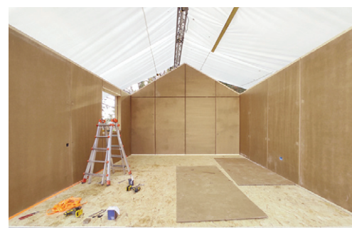
Fig. 2 | Detail of the prototype of a T-Box prefabricated housing unit in corrugated cardboard made with PACOTECH™ port structural load-bearing panels (credit: Archicart®, 2018).
