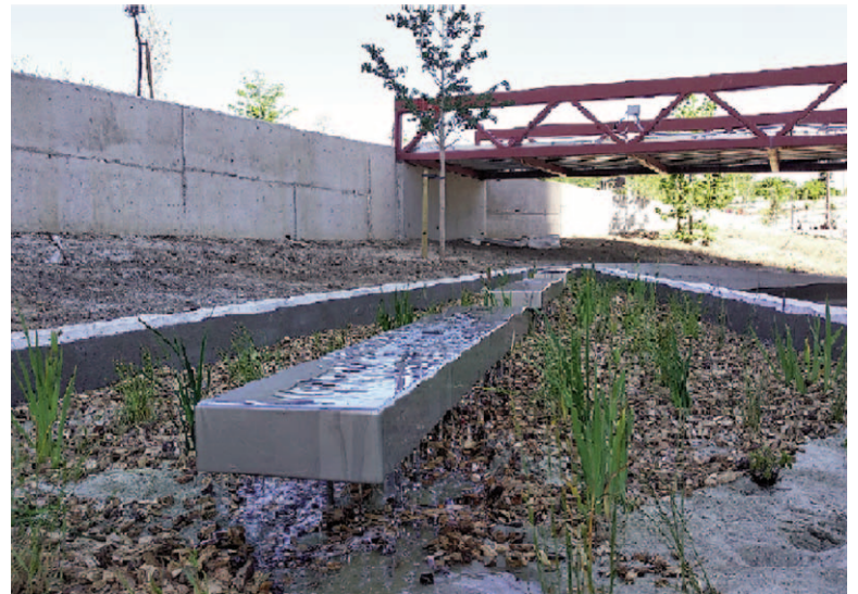
Fig. 2 | The model represented is from the Bluebloqs Circular Water Systems Demonstration project that was installed in the Caledido Park in Madrid, in collaboration with the Universidad Politécnica de Madrid and the Madrid City Council. It is a European project funded by the EIT Climate KIC that seeks to capture, purify and reuse rainwater in cities, creating water reserves within the urban fabric (source: fieldfactors.com, 2022).
