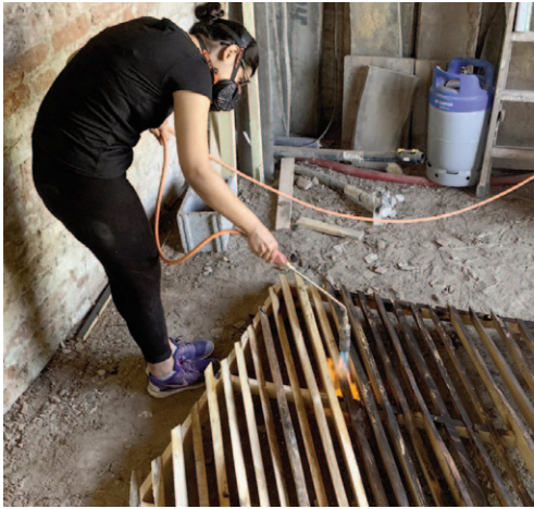
Fig. 7 | VQC: The controlled pre-combustion process of the external envelope panels (credit: Valldaura Labs, 2020).
