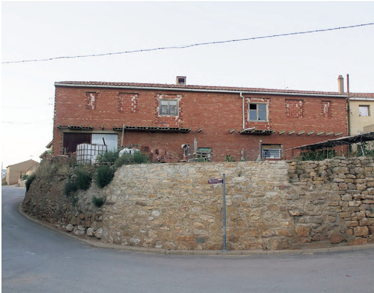
Fig. 6 | Indefinitely unfinished house in Celadas (credit: J. Baró, 2019).
