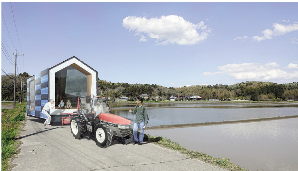
Fig. 13 | EcoCabin, covered in removable transparent photovoltaic panels (credit: S. Tajima, 2020).
