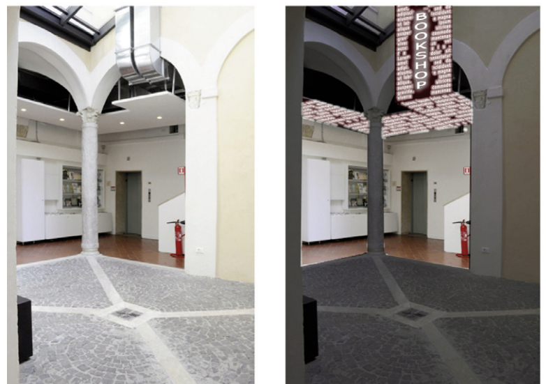
Fig. 7 | Internal courtyard of the Galleria D'Arte Moderna in Rome. Proposal for the application of false ceiling panels, made of an aluminium frame and covered by a textile weft interwoven with optic fibre, lighted with LEDs. The texture forms a customized pattern (in this case, written text) so to increase information related to additional services (graphics by F. Romagnoli, 2020).
