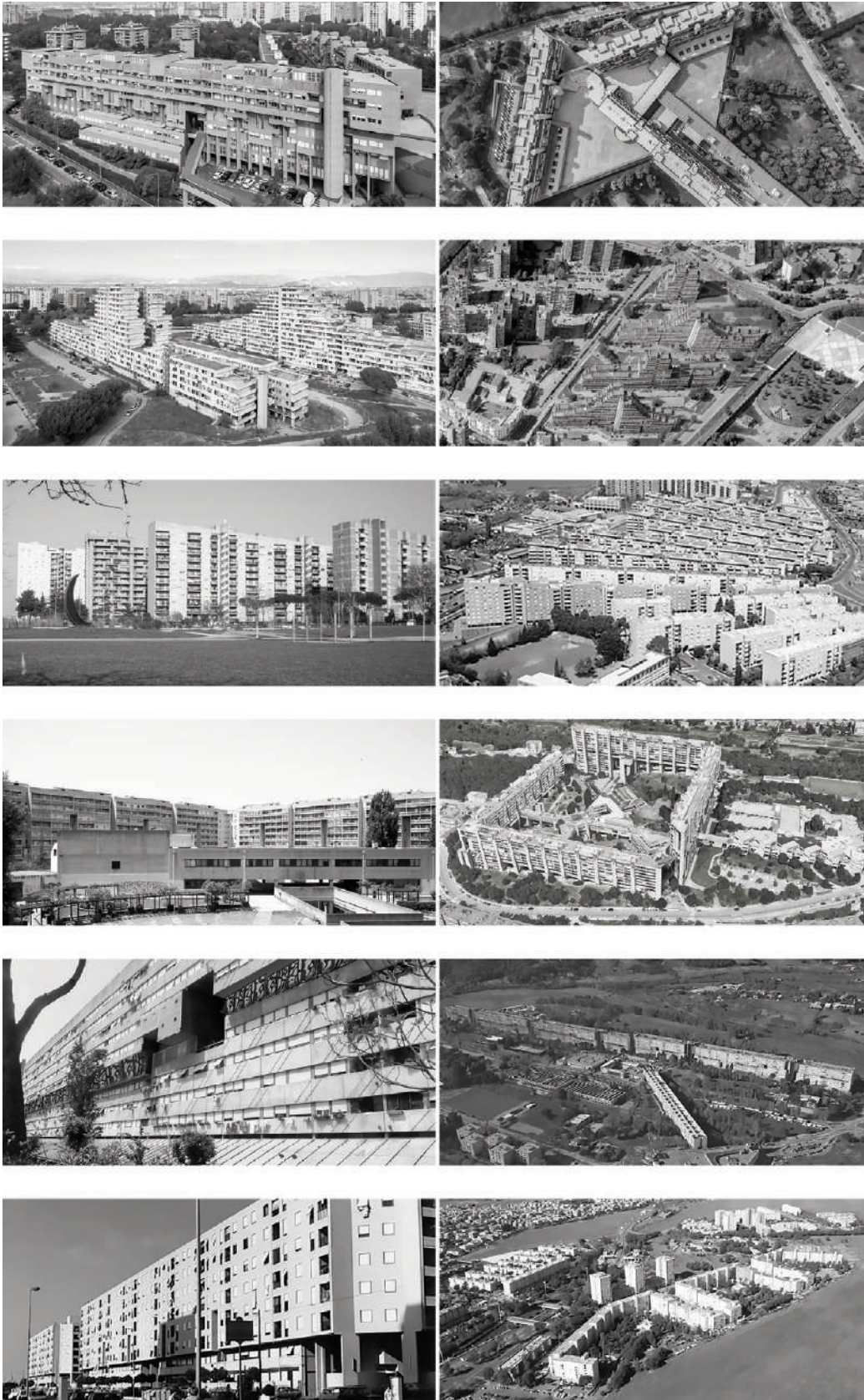
Fig. 3 | The Megaforms housing of Italian 'domesticity': 'Galleratese Quarter, Monte Amiata Housing' in Milan by A. Rossi and C. Aymonino, 1967-1974; 'Vele Scampia' in Naples by F. Di Salvo, 1962-1975; 'Casilino Quarter' in Rome by L. Quaroni, 1965-1974; 'Rozzol Melara Quarter' in Trieste by C. Celli, L. Celli and D. Tognon, 1968-1982; 'Corviale' in Rome by M. Fiorentino, 1975-1984; 'Tor Bella Monaca' in Rome by P. Barucci, 1980-1983 (credits: Daniel Annenkov, Vulcanica Architettura, MIBAC, Kallipolis, Repubblica, Acer, Italiasera).
