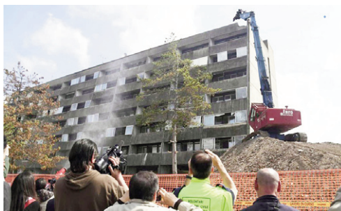
Fig. 12, 13 | Residence Garibaldi 2: the renovated block 3; the demolition of blocks 4, 5 and 6 to be replaced with trees, a basketball court and a children's play area (credits: Comune di Calderara di Reno, courtesy of P. Zullo, 2019; Photo Schicchi, 2019).
