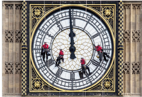
Fig. 7 - Big Ben Clock in London, under continuous maintenance (credit: UK Parliament/Stephen Pike).
