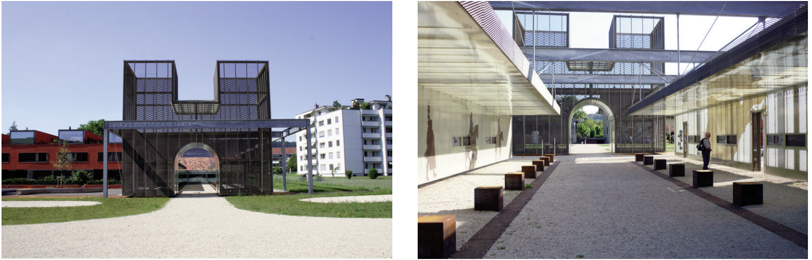
Fig. 19, 20 - Protective shelter and reconfiguration of the Porta and via Pretoria of the Roman town of Vindonissa, in Windisch, Switzerland, designed by Peggy Liechti, Lukas Zumsteg and Adreas Graf in 2007 (credit: Tricoli, 2011).
