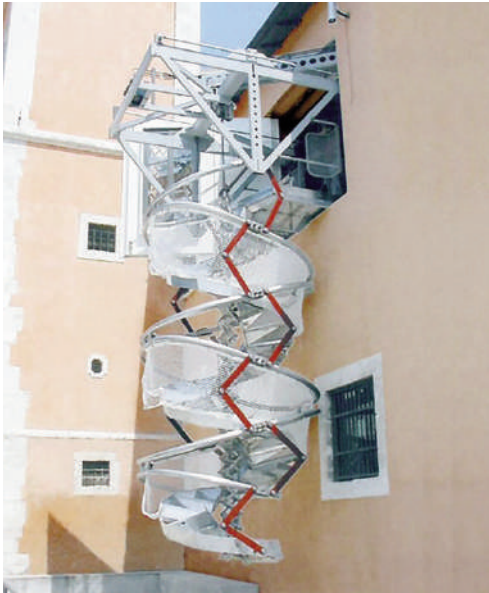
Fig. 5 | Legislative requirements for safety in historic buildings: helioidal retractable staircase (credit: design by Nucleo, Vegaprogetti and Cip – TO; production by Borini Engineering, 2003).
