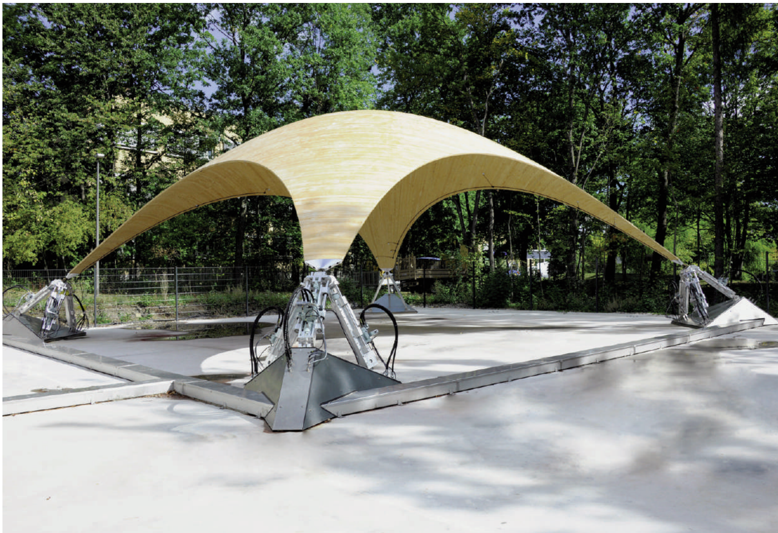
Fig. 2 | Institute for Lightweight Structures and Conceptual Design (ILEK) and Institute for System Dynamics (ISYS), SmartShell, University of Stuttgart, 2012 (credit: ILEK – University of Stuttgart).
