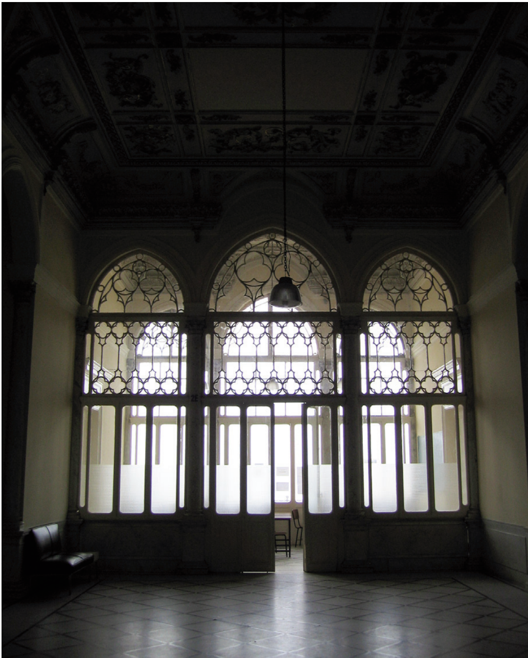
Fig. 9 | Traditional three-arched loggias in Beirut (Lebanon) allow the creation of multifunctional spaces with filtered light, depending on the time of year and needs (credit: X. Casanovas).
