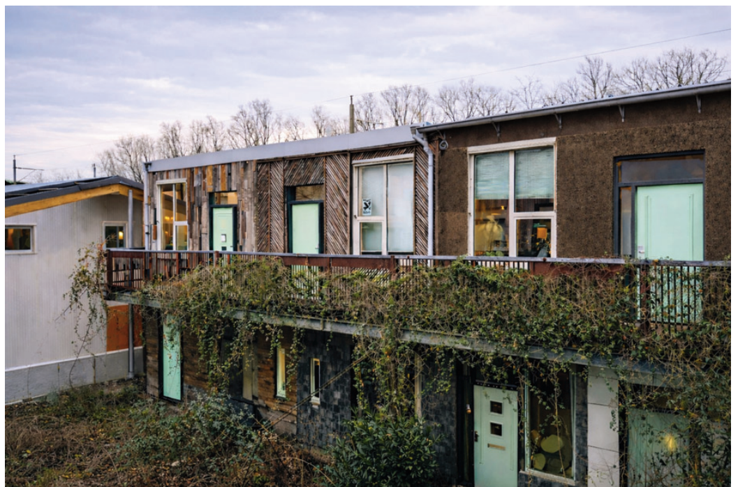
Fig. 11 | Rear façade of Spoor pavilion within 'Het Hof van Cartesius', the two-storey studio strip with reused cladding systems and a continuous balcony, where climbing vegetation forms a green buffer between indoor workspaces (credit: the Authors, 2025).
