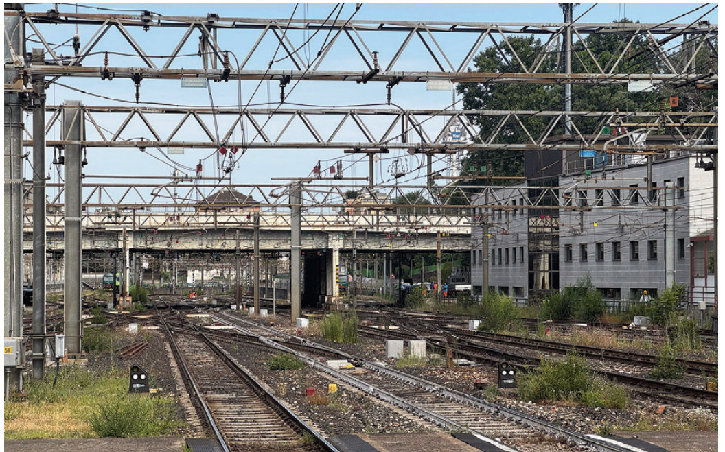
Fig. 8 | Milano Cadorna station and adjacent station building: current state (credit: M. P. Vettori, 2026).
