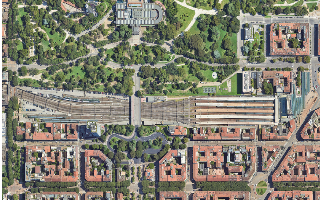
Fig. 6, 7 | Aerial views of the Milano Cadorna station (credits: Google; M. P. Vettori, 2026).
