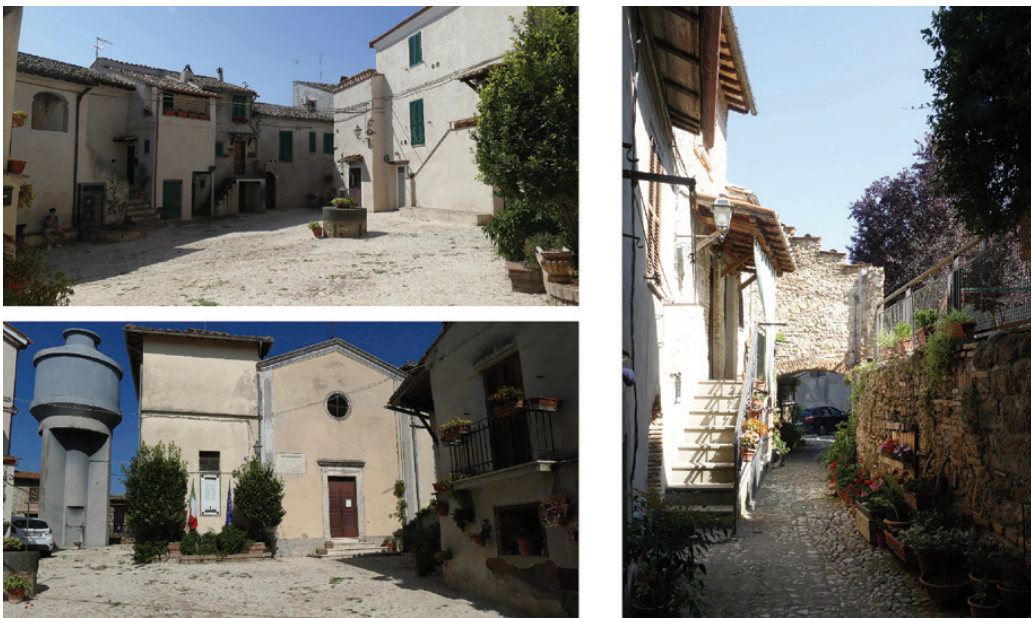
Fig. 9 | Borgo di Cicignano: the square, the Church of Saints Peter and Paul, and the circular pathway connecting the spaces of the borgo (credit: A. Mezzalana, 2024).
