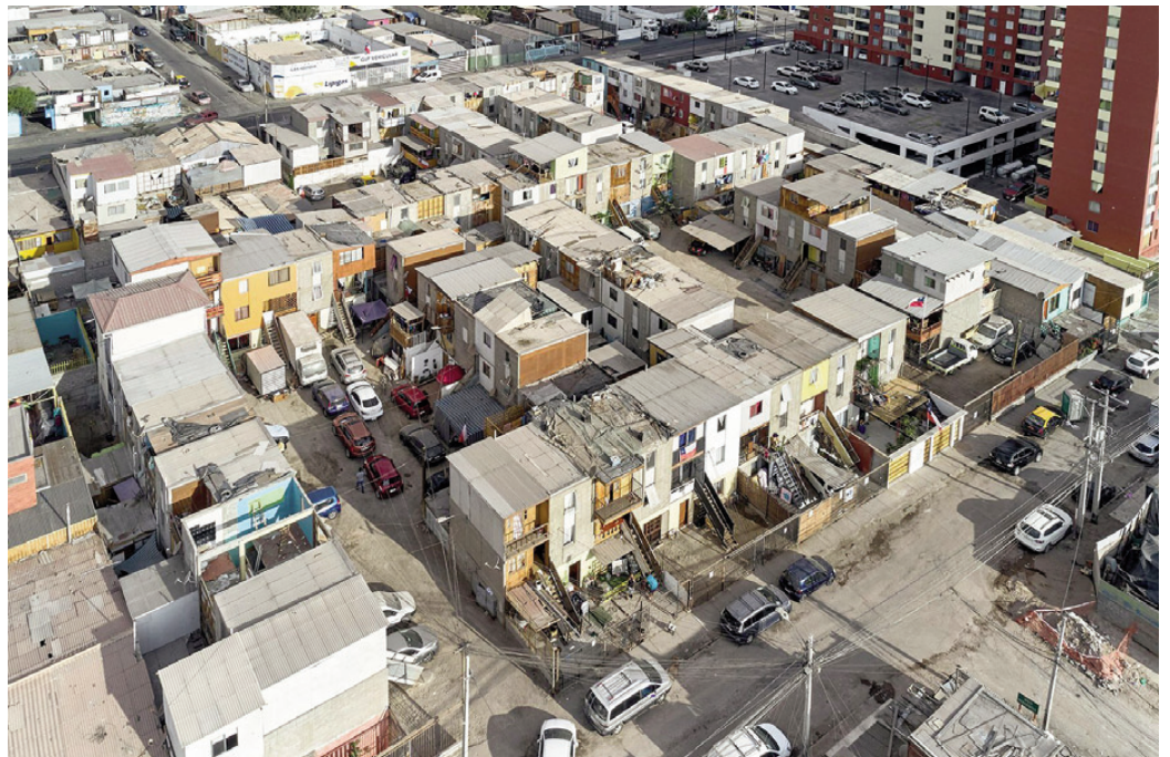
Fig. 2 | Quinta Monroy residential building in Iquique, the 2,500 half-houses built by 2016 (2004), designed by Alejandro Aravena (source: dezeen.com, 2026).
