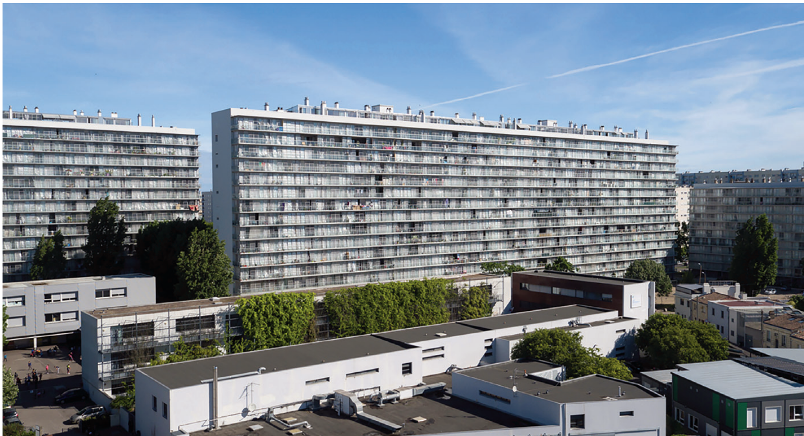
Fig. 6 | The transformation of 530 homes in Bordeaux, extended façades with enclosed balconies (2017), designed by Lacaton & Vassal Architectes, Frédéric Druot Architecture, and Christophe Hutin Architecture (source: archdaily.com, 2026).
