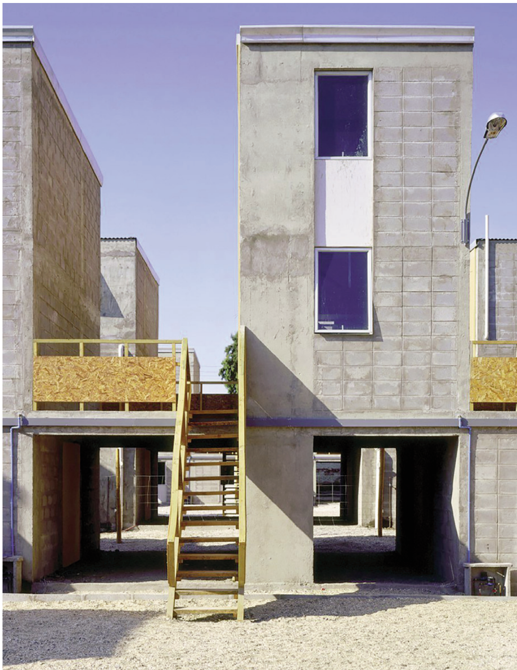
Fig. 1 | Quinta Monroy residential building in Iquique, the half-house structure provided to residents (2004), designed by Alejandro Aravena (source: dezeen.com, 2026).
