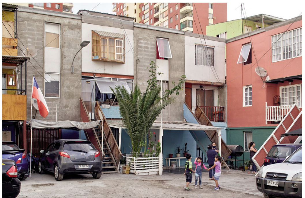
Fig. 3 | Quinta Monroy residential building in Iquique, the half-house structure completed by the residents (2004), designed by Alejandro Aravena (source: dezeen.com, 2026).
