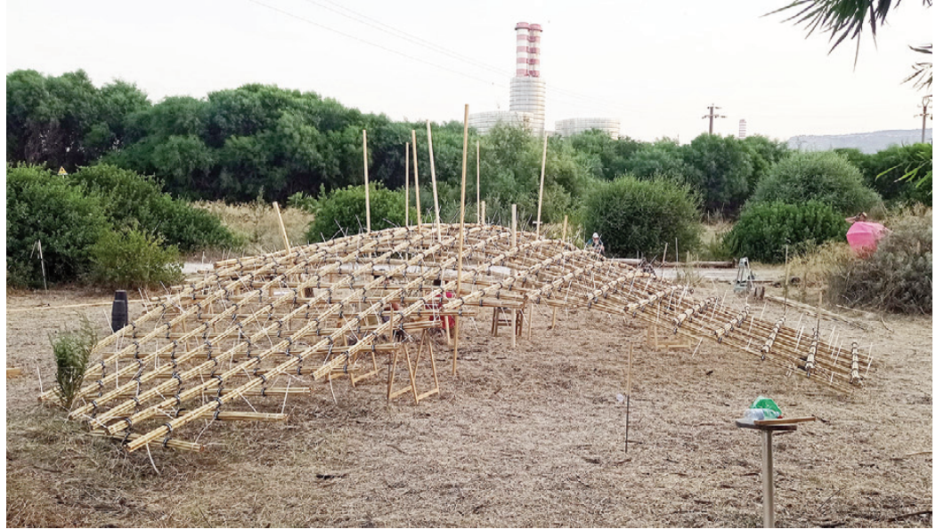
Figg. 13, 14 | Images of the assembly phases of the educational room structure (credits: the Authors, 2025).
