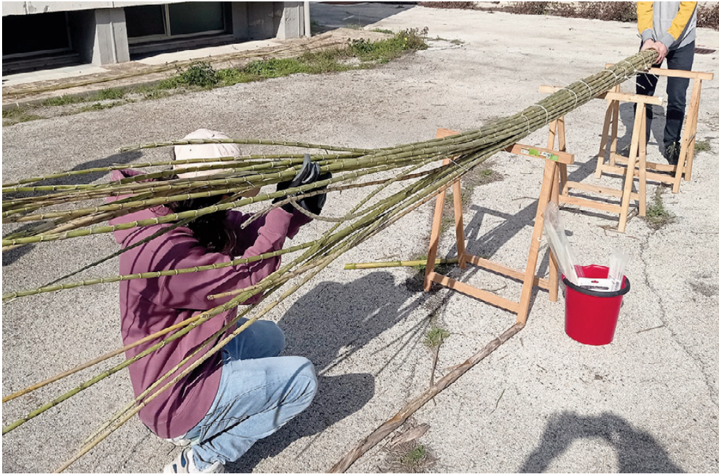
Figg. 7, 8 | Images of several preparation phases of the bundles composing the structural system (credit: the Authors, 2025).
