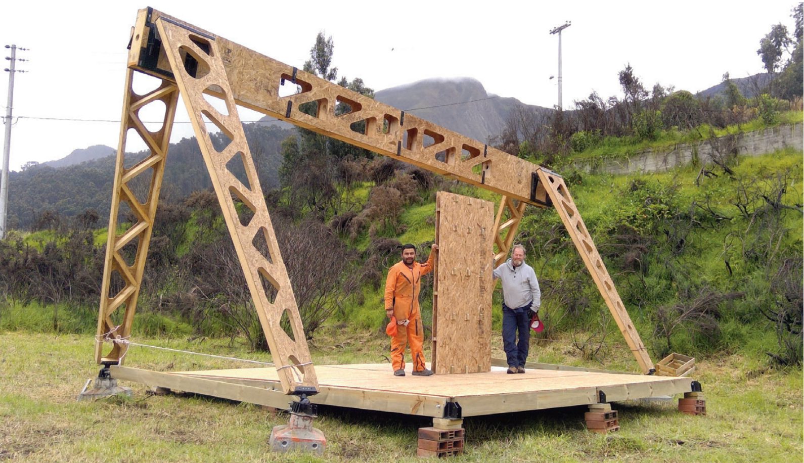
Fig. 15 | Prototype construction on rural setting in Suesca, Cundinamarca (credit: C. Nieman and D. Velandia 2024).
