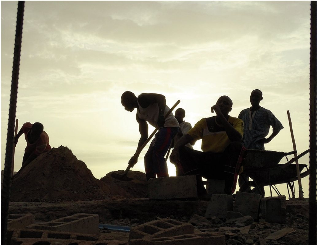
Fig. 15 | Workers during the construction of the Toumoumba barrage (credit: the Authors, 2018).
