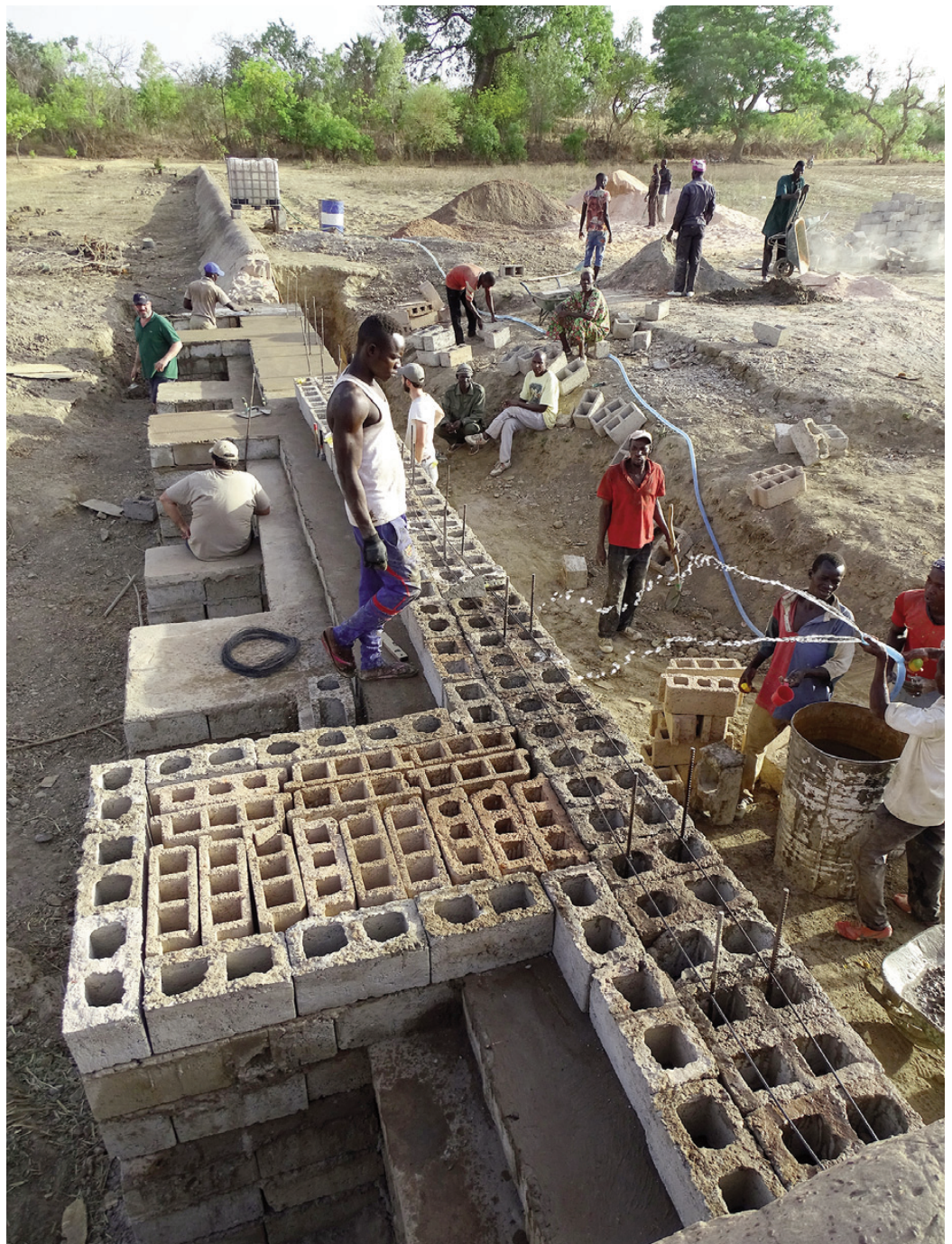
Fig. 10 | The Toumoumba barrage under construction (credit: the Authors).
