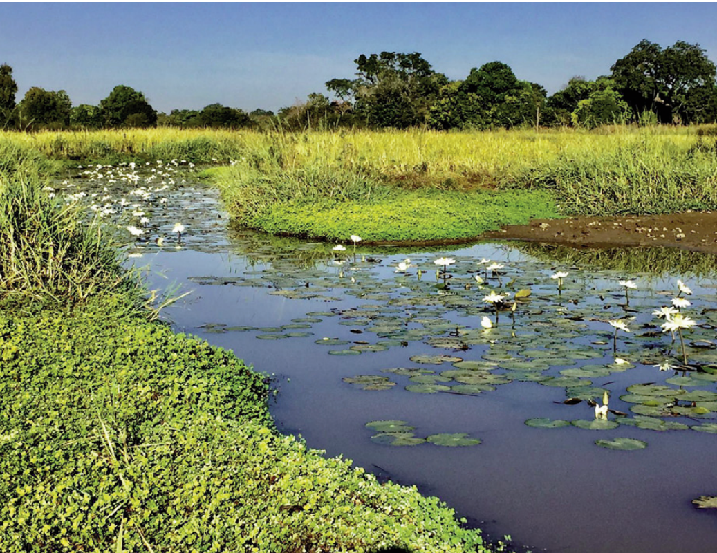
Fig. 11 | The Toumbouba barrage after restoration (credit: the Authors).
