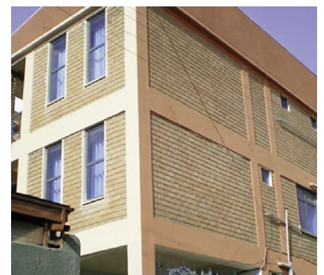
Fig. 2 | Traditional solution 1: load-bearing walls in stone-cut blocks (credit: the Authors, 2025).
