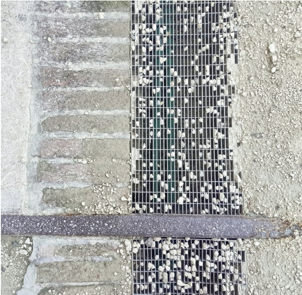
Fig. 6 | A pavement segment revealing the complex coexistence of various materials, including iron, bricks, gravel, and stabilised earth, illustrating the diverse engineering practices utilised in urban surface construction (credit: T. Moretto, 2025).
