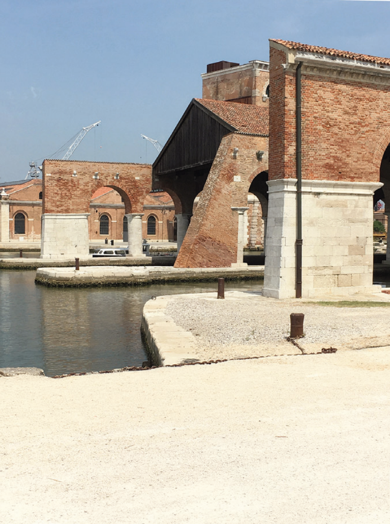
Fig. 4 | Spatial configuration of the Gaggiandre shipyards in relation to the condition of the adjacent pavement (credit: E. Sorbo, 2025).
