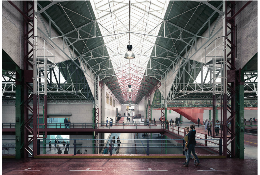
Fig. 15 | KANAL in Brussels (2018-2025), designed by Sergison Bates architects: the transformation of the former Yser Citroën factory in downtown Brussels as a centre for modern and contemporary arts (credit: Sergison Bates architects, 2018).
