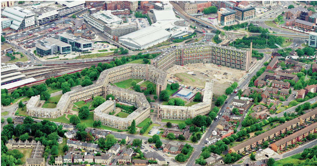
Fig. 12 | Park Hill Estate, Sheffield: building life was extended by reinforcing and rejuvenating the structure, while the infill was renovated using adaptable and moveable design (source: hoddereducationmagazines.com).
