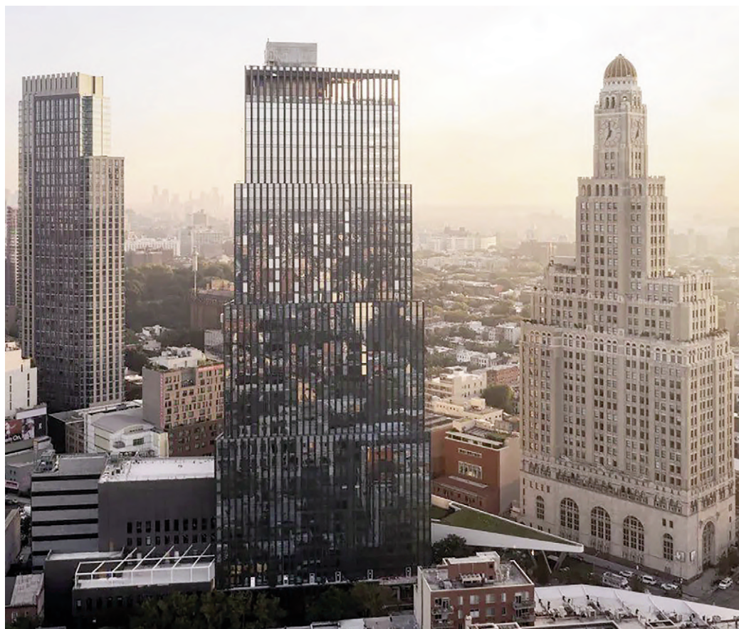
Fig. 4 | 44-storey tower in Brooklyn, New York City's first all-electric skyscraper (credit: P. Bendov, 2024).
