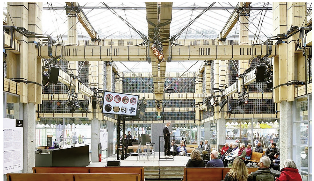
Fig. 13, 14 | Temporary People's Pavilion, Eindhoven, 2017 Dutch Design Week. The structure was made entirely from borrowed materials, while the pavilion was clad in interlocking plastic tiles recycled from PET bottles donated by town residents (source: tudelft.nl; credit: F. Dujardin).
