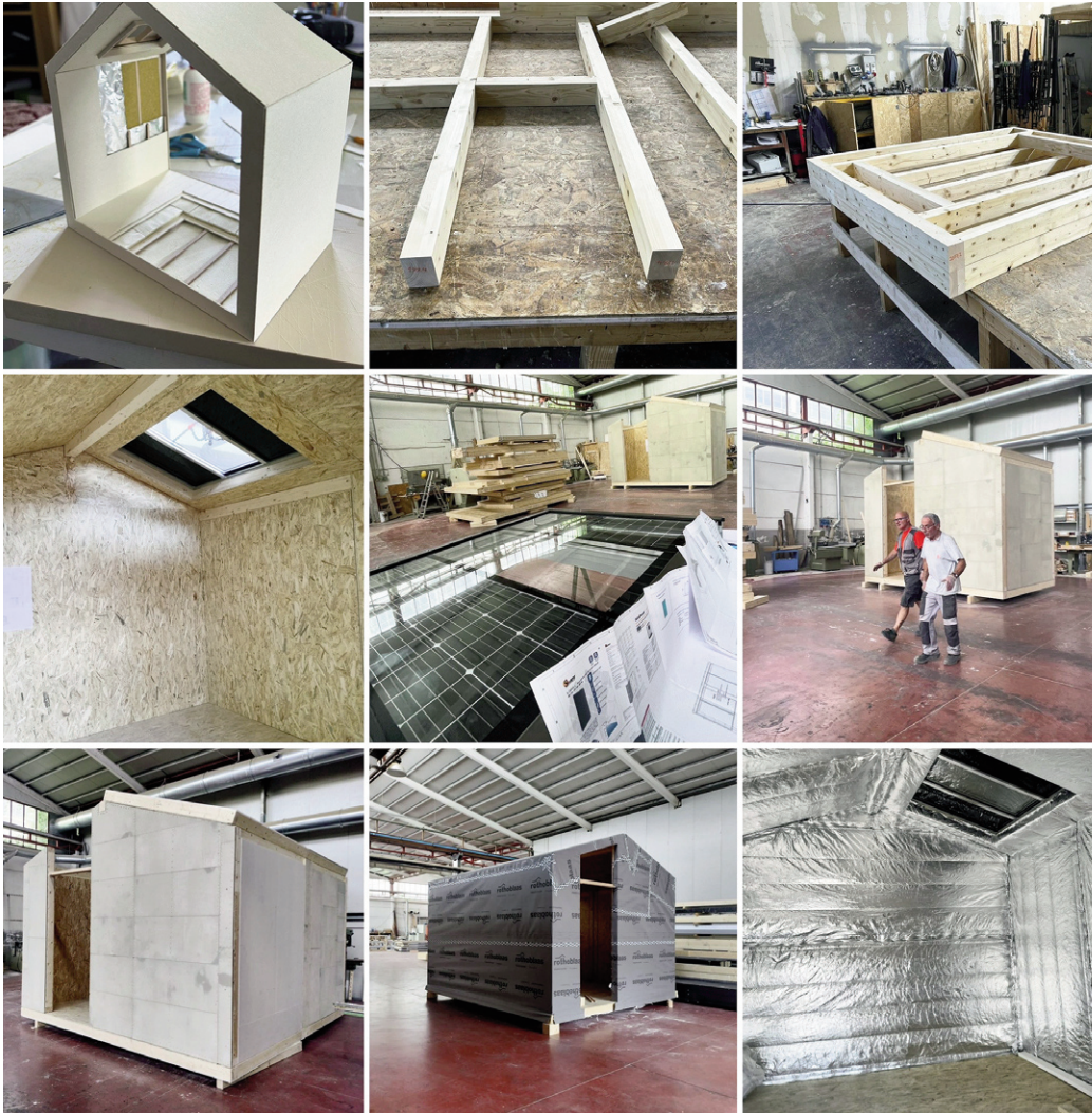
Fig. 14 | Assembly stages of the nZEM Prototype (credit: R. Romano, 2023).
