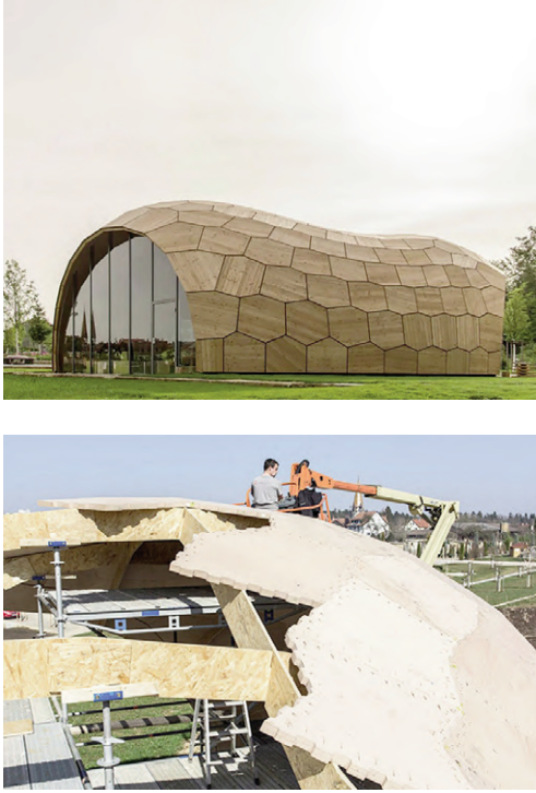
Figg. 1, 2 | Landesgartenschau Exhibition Hall in Stuttgart, designed by Achim Menges and Jan Knippers, 2014 (source: dezeen.com; designboom.com).
