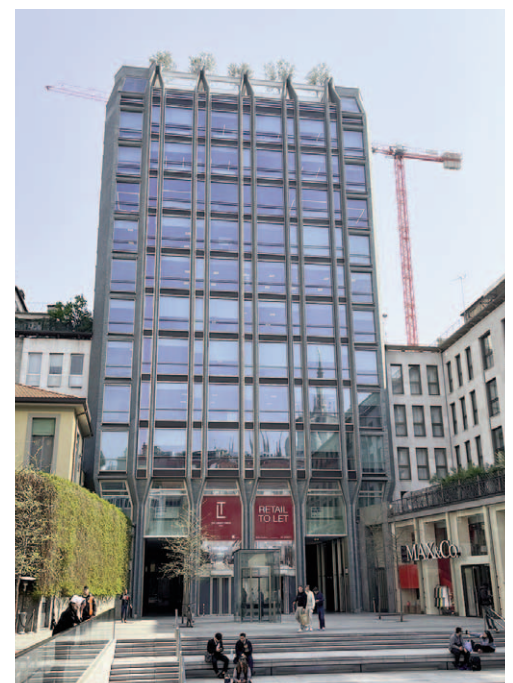
Fig. 13 | Unipol Tower ‘vertical nest’ in Milan, designed by Mario Cucinella, 2016: Green project designed by Marilena Baggio (source: blog.urbanfile.org , 2022).
