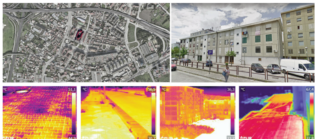
Fig. 1 | Urban setting of the building under study and survey of the environmental and performance characteristics of the context through thermography.
