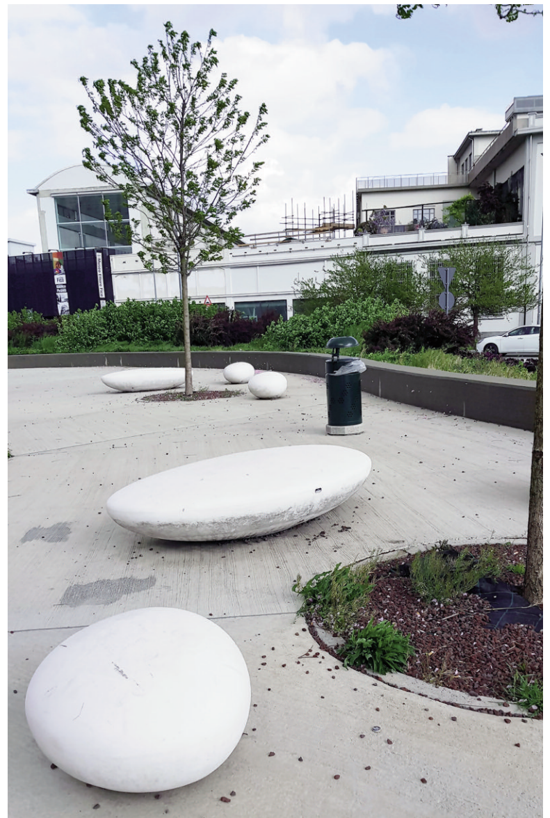
Fig. 3, 4 - Monolith urban furniture benches in Turin, made of concrete containing fine aggregates. On the left (area: Corso Palermo), without superficial finishing: colour variation, patina and local staining, after 4 years operating life; On the right (area: via Cigna), with superficial chromatic finishing: colour variation, patina in lower area, after 3 years operating life (credits: R. Maspoli, 2019).
